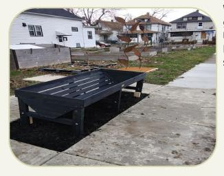
**Knee clearance** underneath the planter should be between 9" and 27", with a maximum depth of 25".
