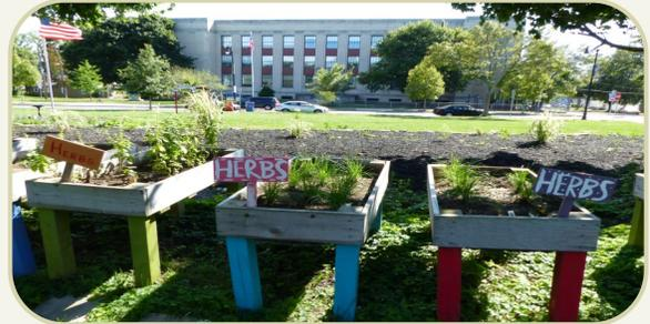
**Knee clearance** underneath the planter should be between 9" and 27", with a maximum depth of 25". Width should be 30" minimum. Minimum depth should be 11" deep at a height of 9", and 8" deep at a height of 27".<sup>3</sup>
