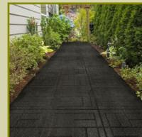
Plastic, open grid systems allow soil, grass, or other plants to fill in flush with the grid system creating a natural looking pathway. The open grid however can be penetrated by canes or other objects if not properly tamped down.<sup>4</sup>
