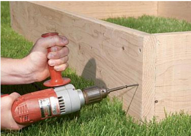
After drilling pilot holes, attach one of the side boards to an end board with three evenly spaced screws.
