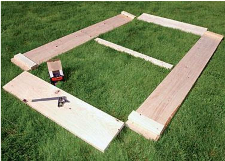
Cut the 2-by-4 board into one 4-foot length, to serve as a center brace, and four 1-foot lengths for corner supports. The two uncut boards will become the sides of the raised bed.
