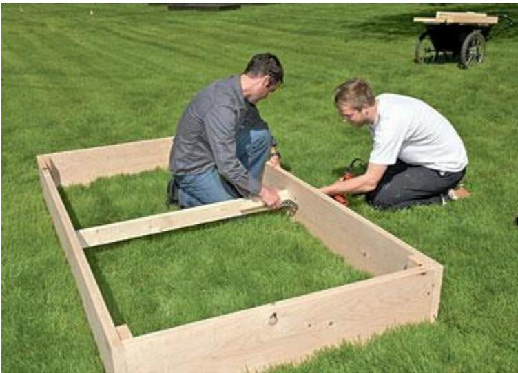
Attach the center brace to join the two sides at their midpoints. Use a square to position the brace at a right angle to the sides (5). The brace prevents the sides from bowing outward when the bed is filled with soil.
