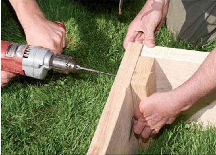
Place one of the corner supports in the angle between the boards and attach it to the side board with three screws. Repeat for the remaining three corners.
